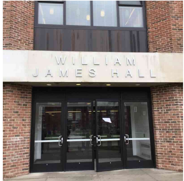
Facade C - West Quad
