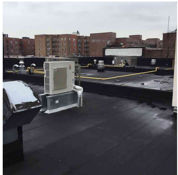
Roof 1 - North view
