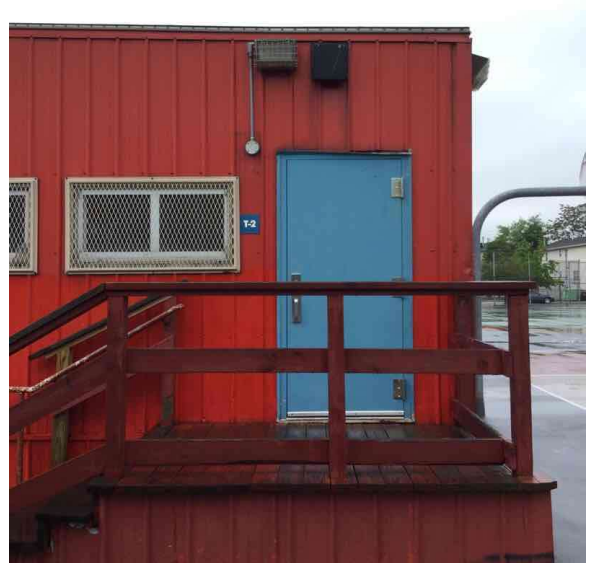
Facade B - T2 Entrance
