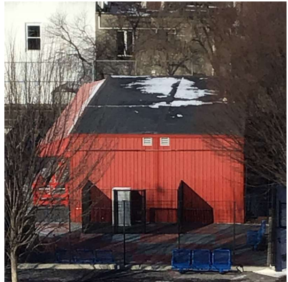
Roof 1 - Northwest View
