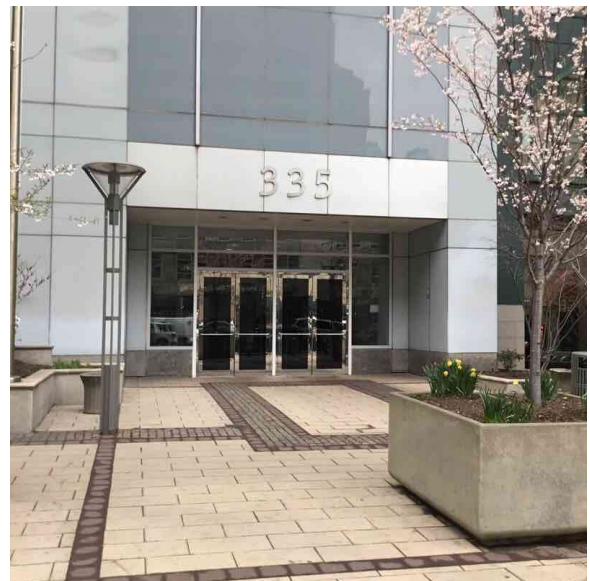
Facade A - Adams Street
