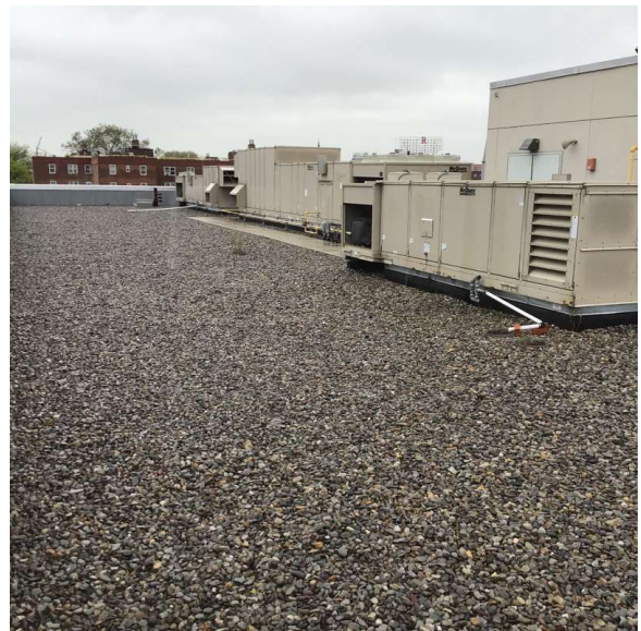
Roof 1 - Northeast view
