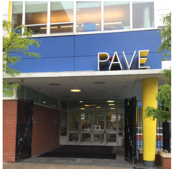
Facade A - Mill Street
