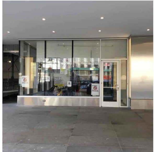
Facade A - Washington Street
