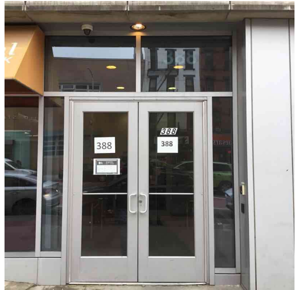
Facade A - West 125th Street
