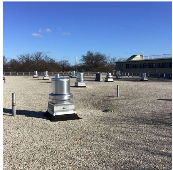
Roof 6 - Northeast view
