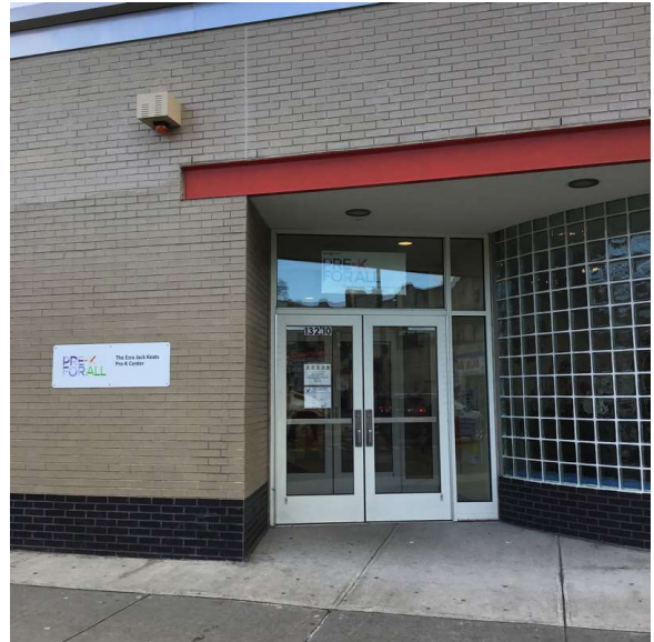
Facade A - Jamaica Avenue
