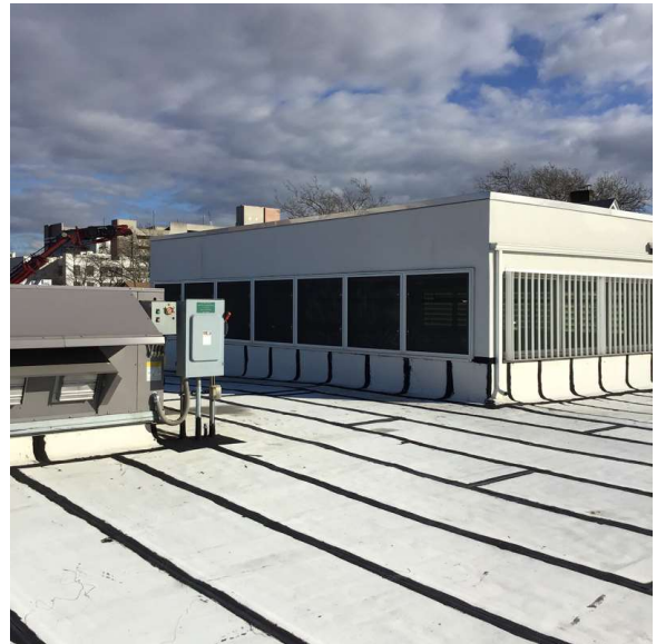
Roof 1 - East view
