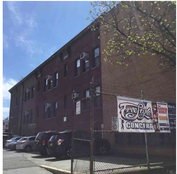
Corner at Myrtle Avenue - South view
