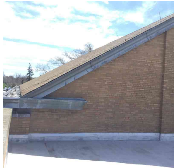
Roof 2 - South view
