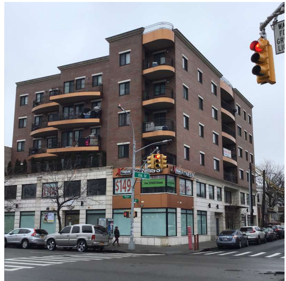
Corner of Northern Boulevard and 106th Street - Southeast View
