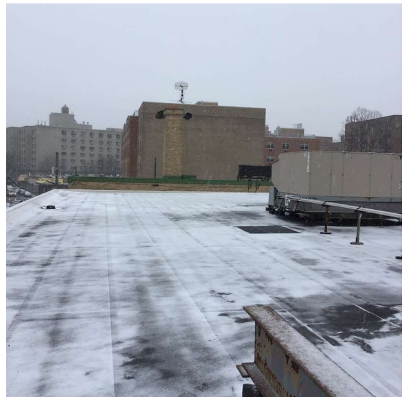
Roof 2 - East view
