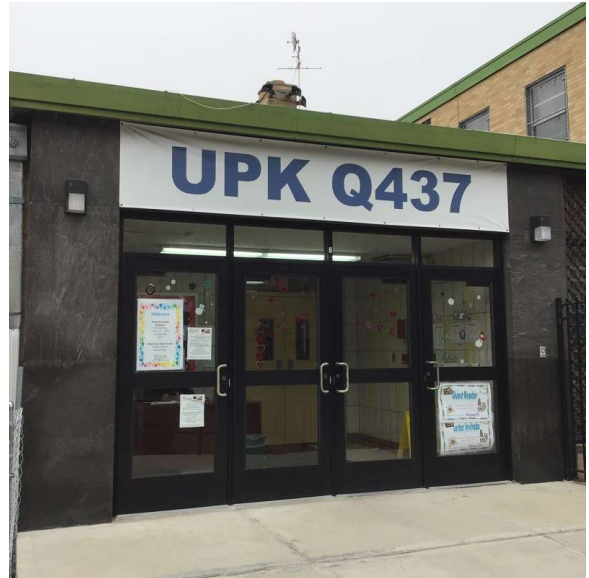
Facade A - 98th Place
