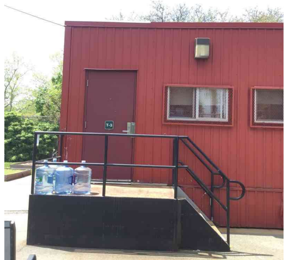
Facade C - 214th Lane
