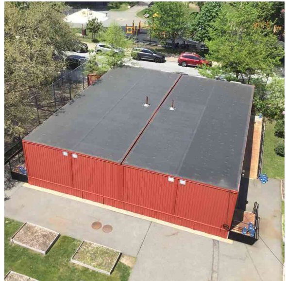
Roof 1 - North view
