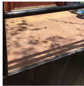
Facade A No violations recorded.
