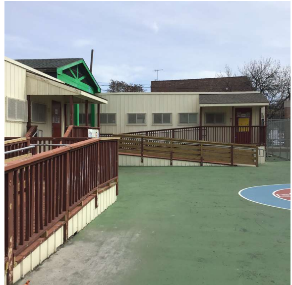
Facade A - Southwest View
