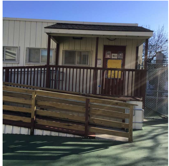
Facade A - Unit T1
