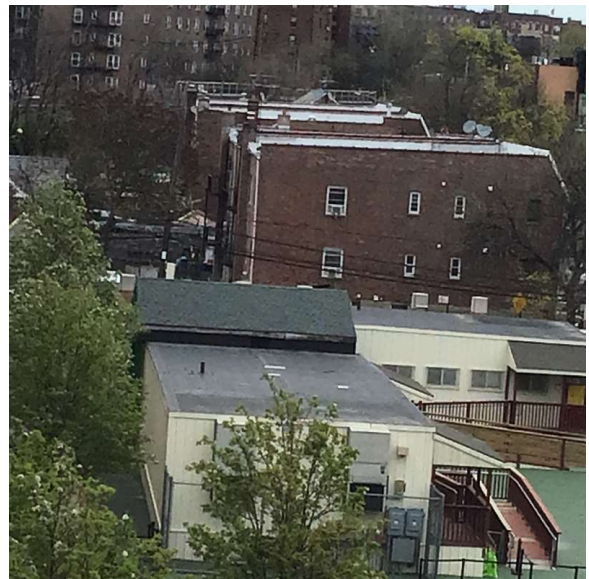
Roofs 2,1 - North View
