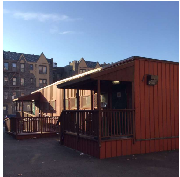
Facade C- South View
