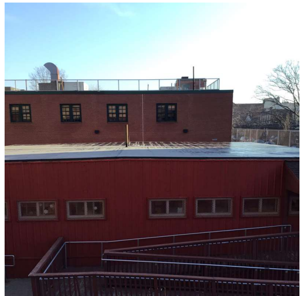
Roof 1- North View
