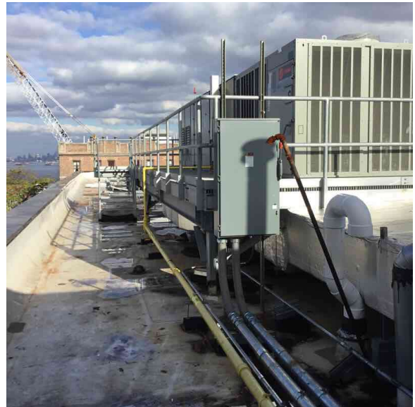
Roof 1 - East view
