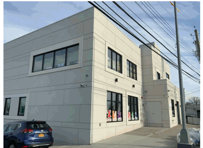
Corner of Cherokee Street and Father Copadanno Boulevard - North View
