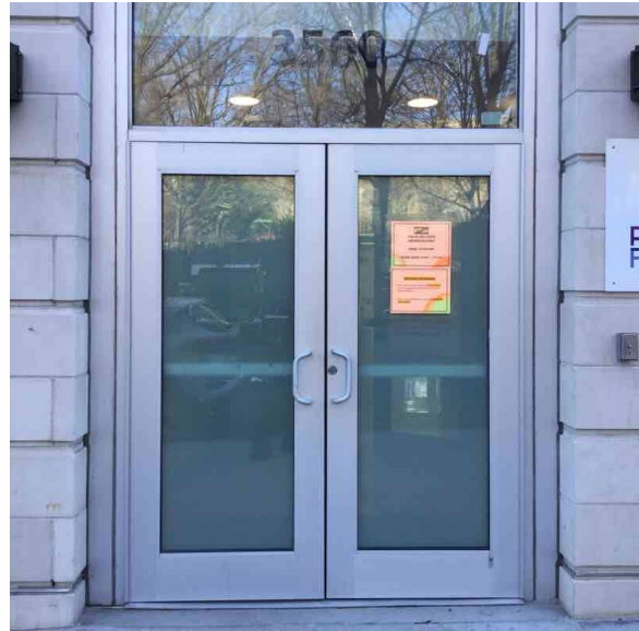
Facade A - Webster Avenue
