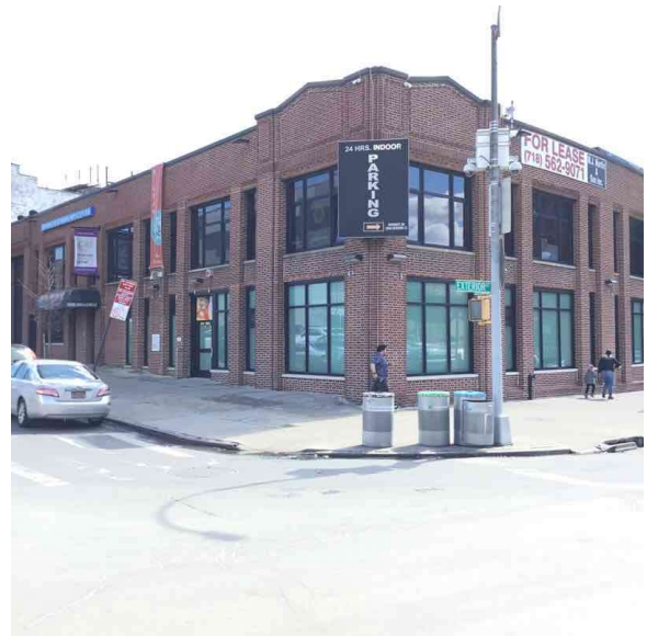
Corner of West 230th Street and Exterior Street - Southwest View
