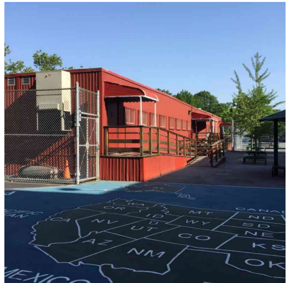
Facade A - Northwest view
