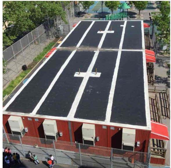
Roofs 1-4 - Northwest view
